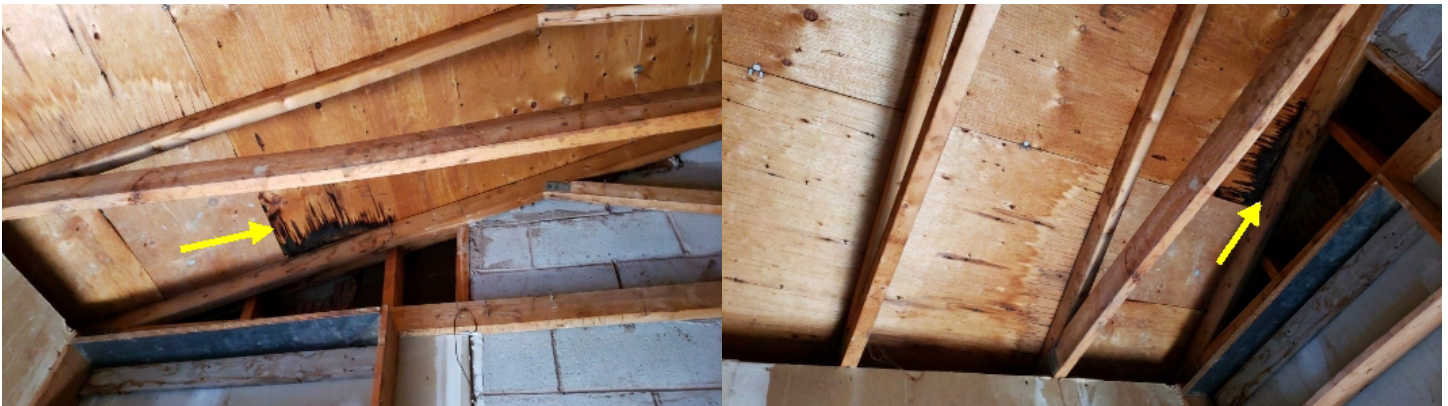
Evidence of past water penetration observed.
