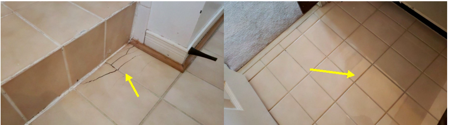
Cracked / Chipped tiles noted.
