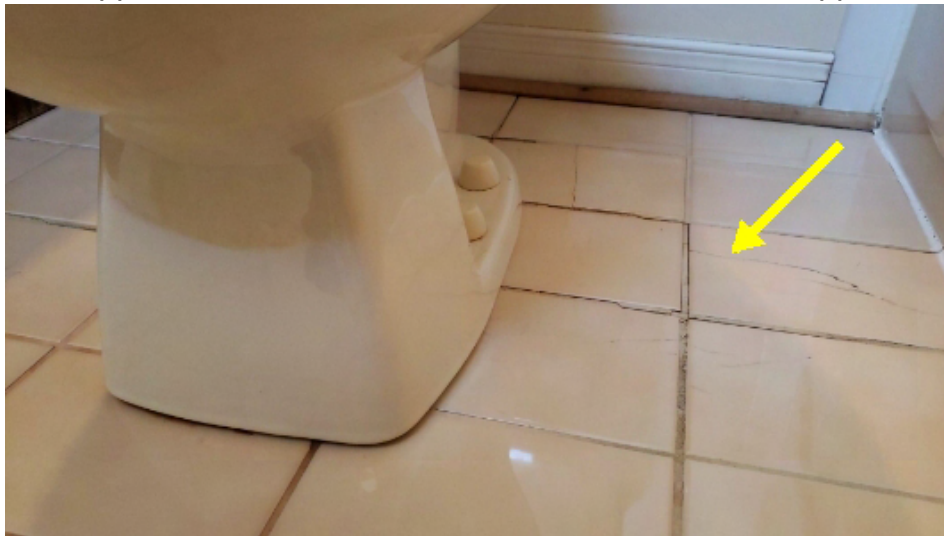
Cracked / Chipped tiles noted.
