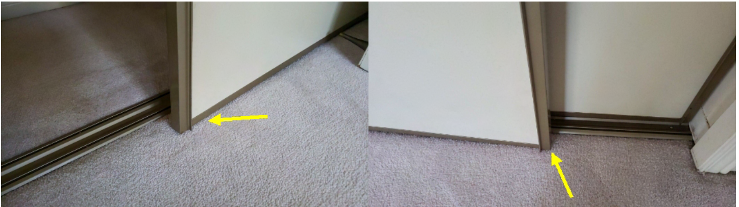
Door does not latch, needs adjustment.
