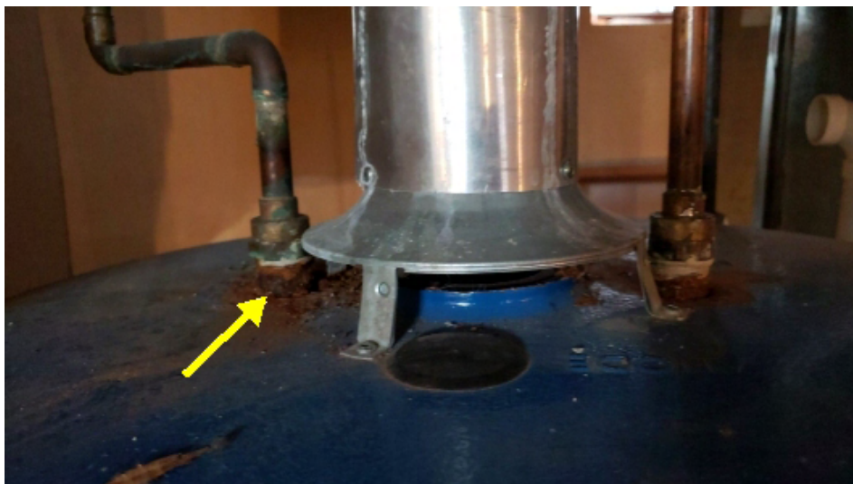
Corrosion noted at fittings.
