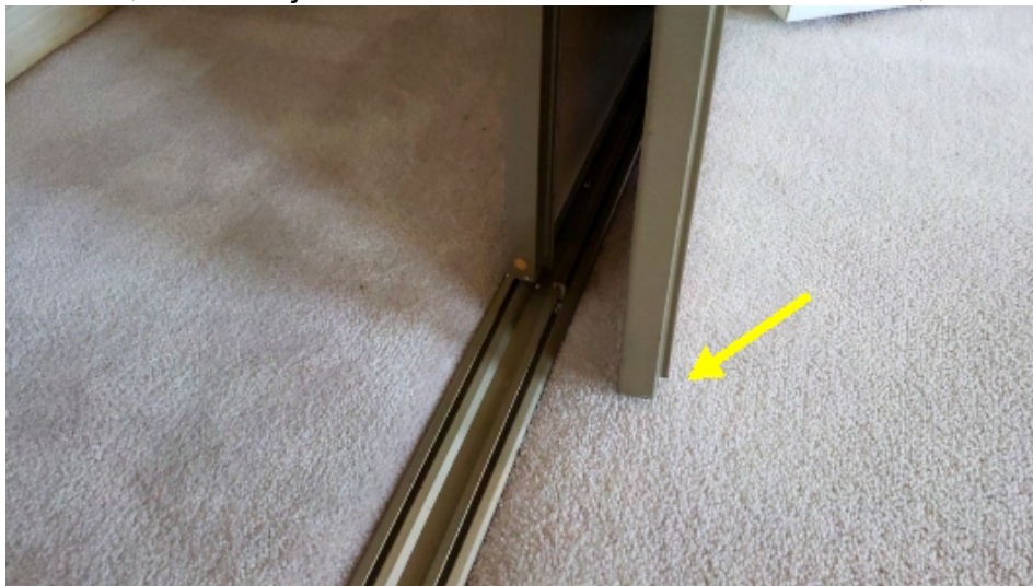
Door does not latch, needs adjustment.
