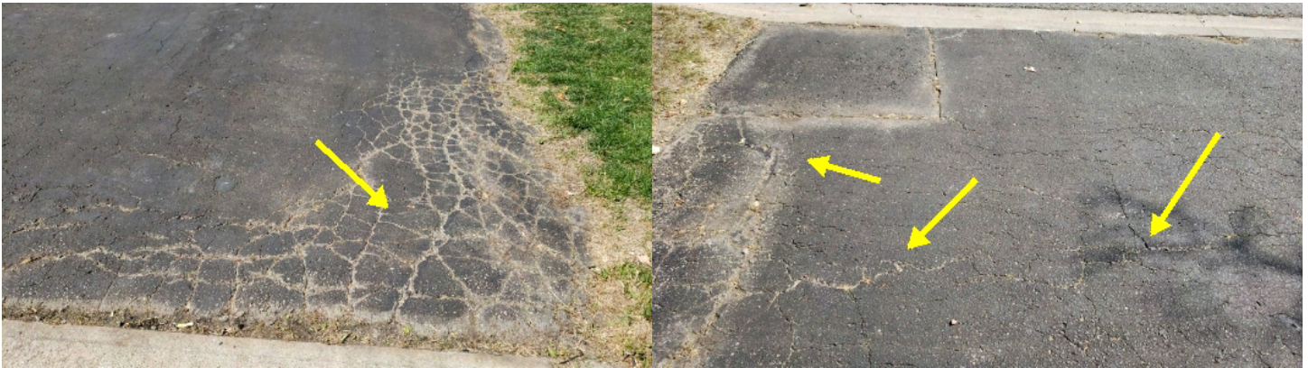
Settlement and common cracking noted.
