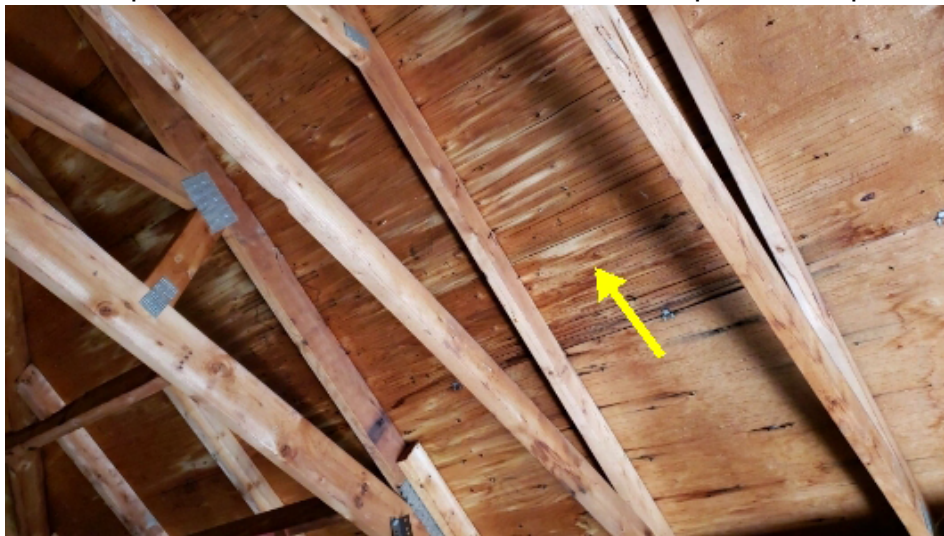
Evidence of past water penetration observed.
