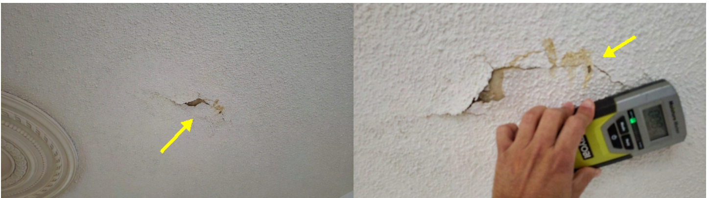
Evidence of past water penetration observed.
