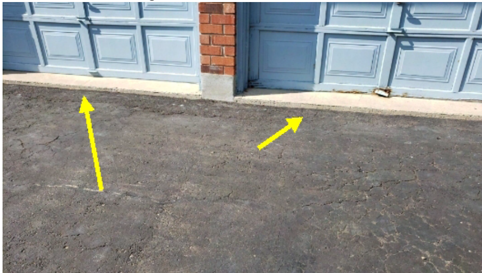
Settlement and common cracking noted.
